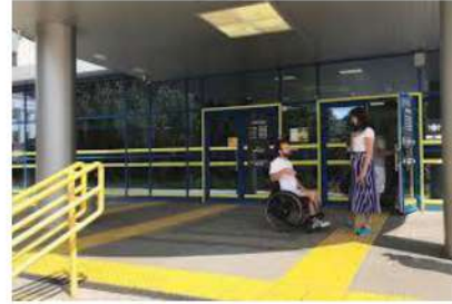
Fig. 2. Accessible pedestrian ramp – example of inclusive environmental design
